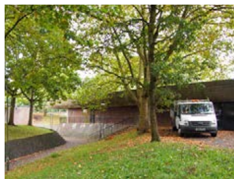
Existing energy centre.
