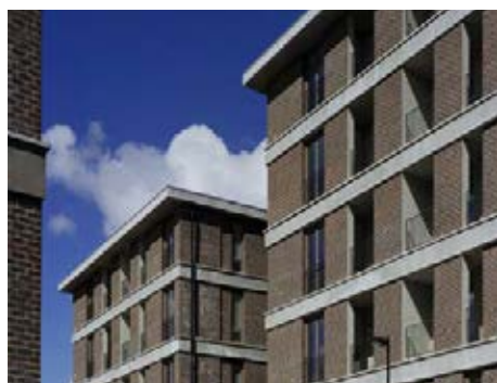
Order and simplicity in facade treatments. Finsbury Park
