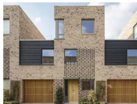
Repetitive building type with terraces. Great Knighton, PTEa.
