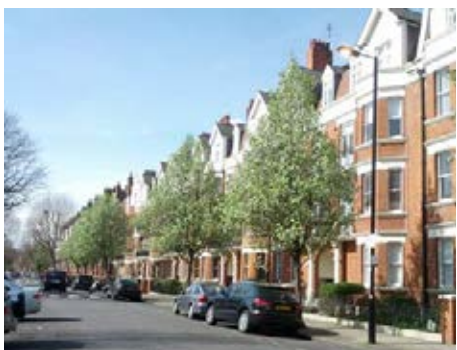
Formal tree lined route with parallel parking and tall repetitive frontages. Maida Vale, London
