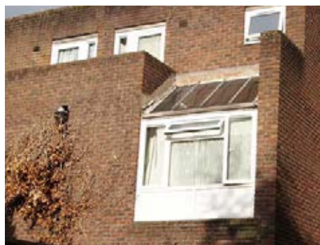
Existing 3 storey townhouse type on site, with 'winter garden' at the rear.
