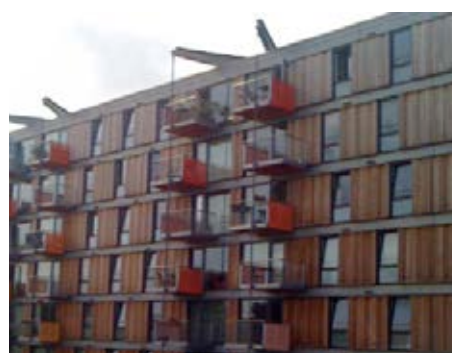
Prominent, lively frontage Adelaide Wharf, Haggerston
