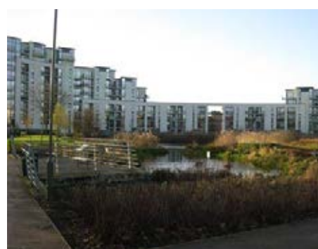
The new development to the west of the park fronting onto a wildlife pond
