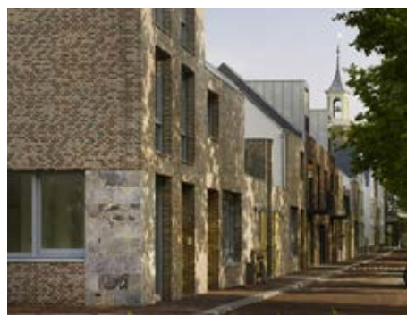
Informal building heights. Molenplien, Netherlands
