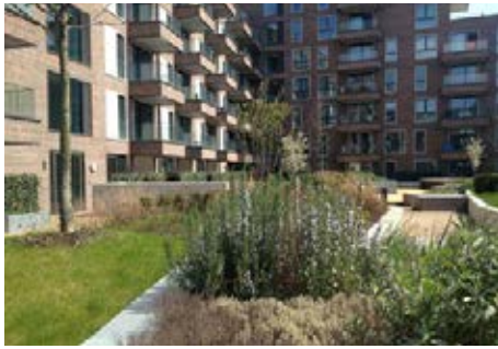
Raised gardens Thames Barrier East Development
