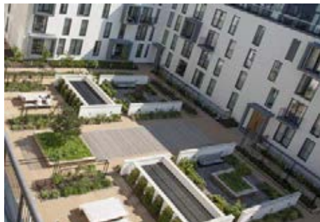
Raised shared courtyard & integrated planting Podium at Bath Western Riverside
