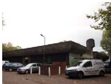
Existing energy centre.
