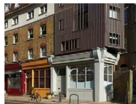
An active ground floor level. Alex Monroe Studios, Southwark
